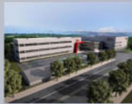
EMS ADC Suzhou Under Construction 苏州艾曼斯ADC动工
